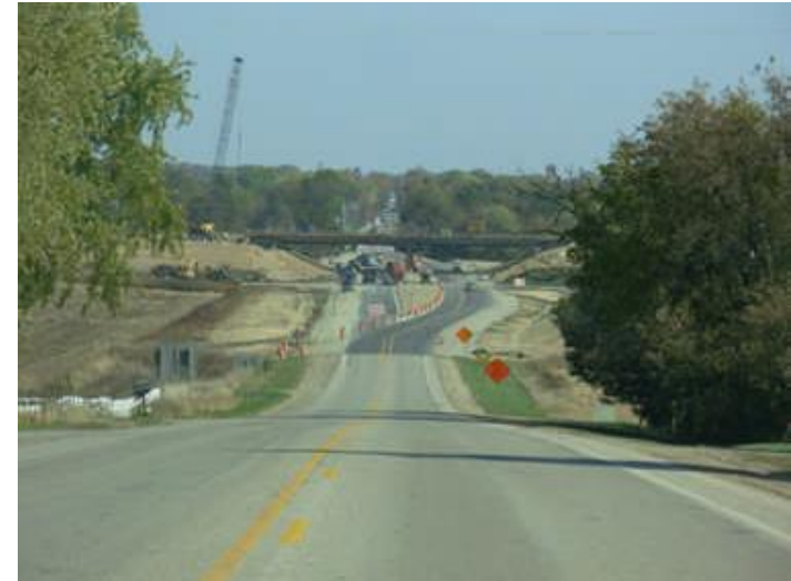
The WIS 26 bypass around the City of Jefferson when it was under construction in 2009.
